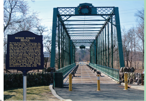
Nevius Street Bridge
