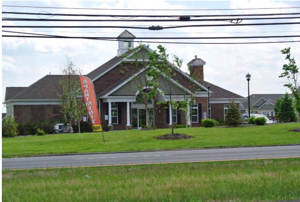
Stone Bridge at Raritan
