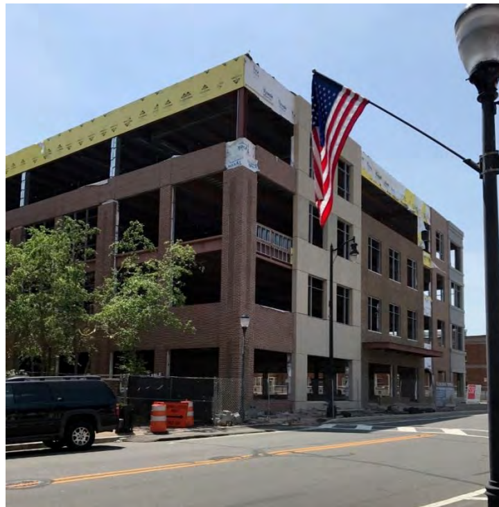
Somerville Commons redevelopment project under construction, May 2017
