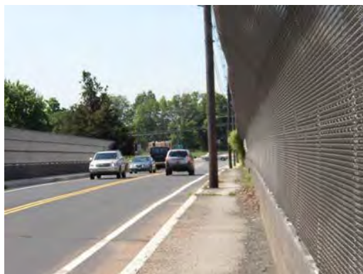
Arterial Road, North Bridge Street, Bridgewater
