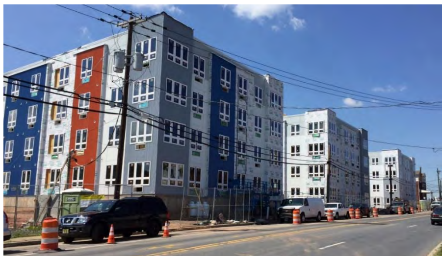
Cobalt Apartments in Somerville under construction in 2016
