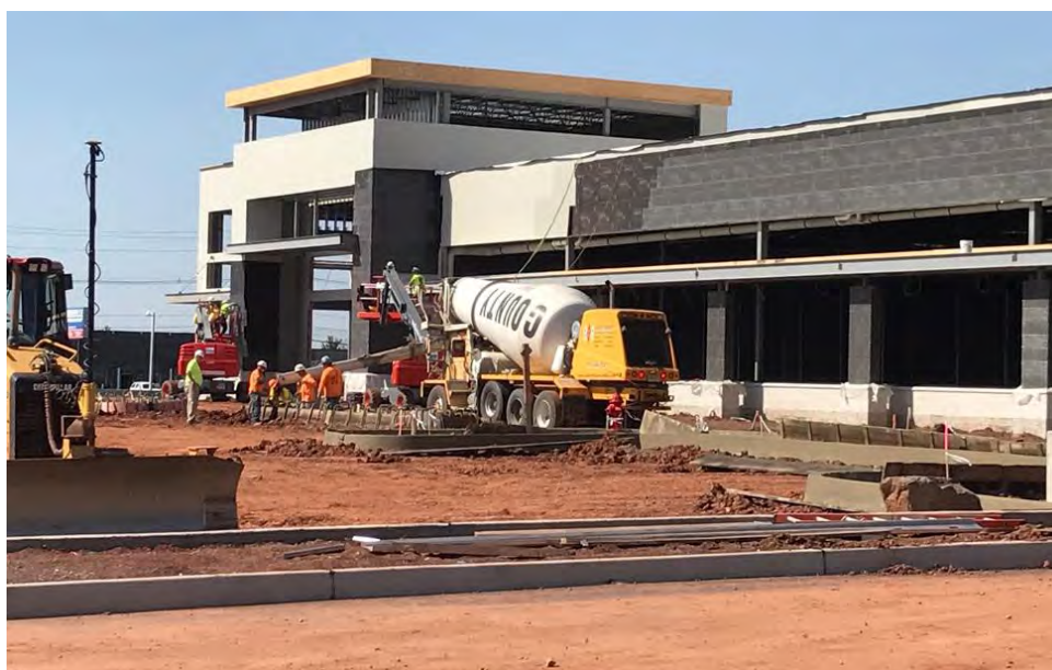
Chimney Rock Crossing West under construction in April 2017
