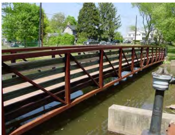
Raritan Power Canal Pedestrian Bridge
