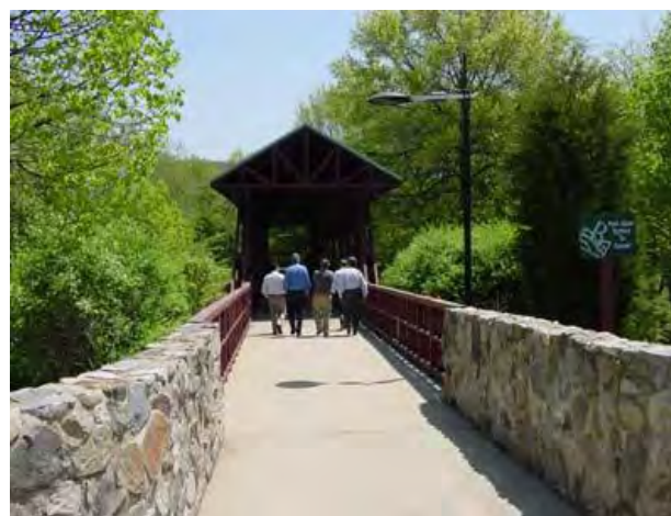
Pedestrian Walkway, Bridgewater
