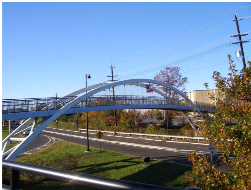
Sgt. Andrew Lobosco Pedestrian Bridge, Somerville - Bridgewater
